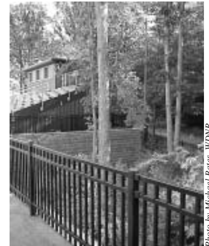
Retaining walls are used to maintain original grade and protect roots of mature trees.
