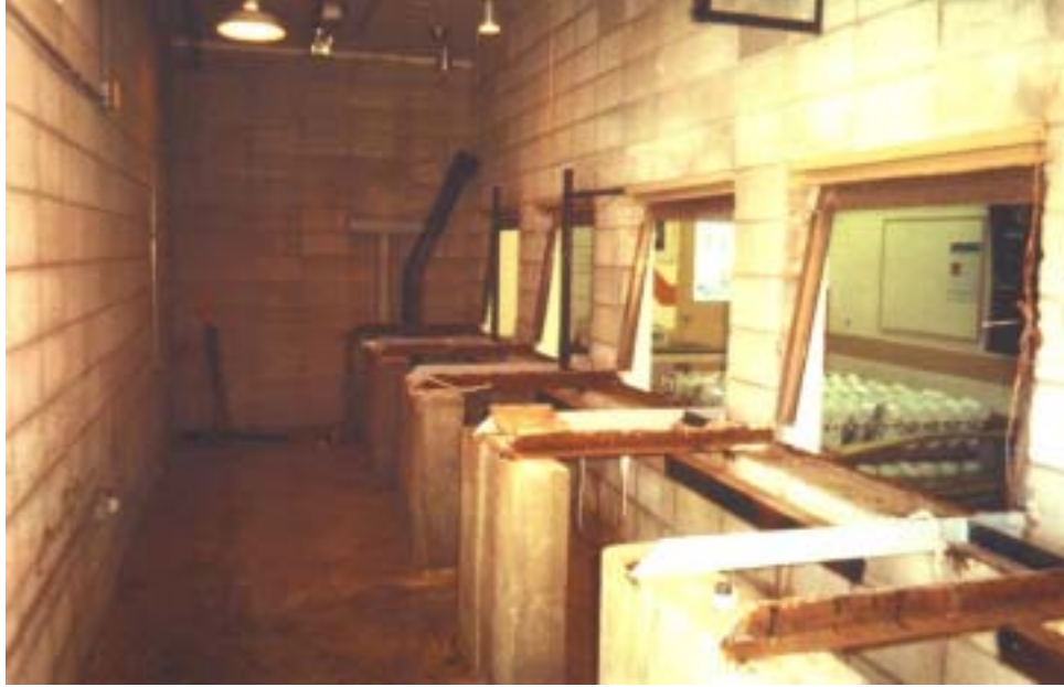
Figure 4. Cement wall that housed viewing tanks.
