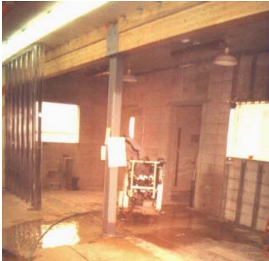
Figure 5. Wooden support beam.
