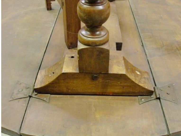
Figure 4. Detail of butterfly hinges, Gate-leg trestle table. Probably New York, c. 1660-1700. Soft maple, maple, butternut, cherry, oak. 1958.0527. Gift of Henry Francis du Pont, Winterthur Museum. Photo by author, 2014.
